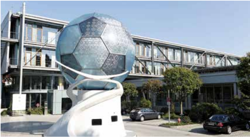
... AND AS THE IDENTIFYING FEATURE OF DFB HEAD OFFICE IN FRANKFURT'S CITY FOREST.
